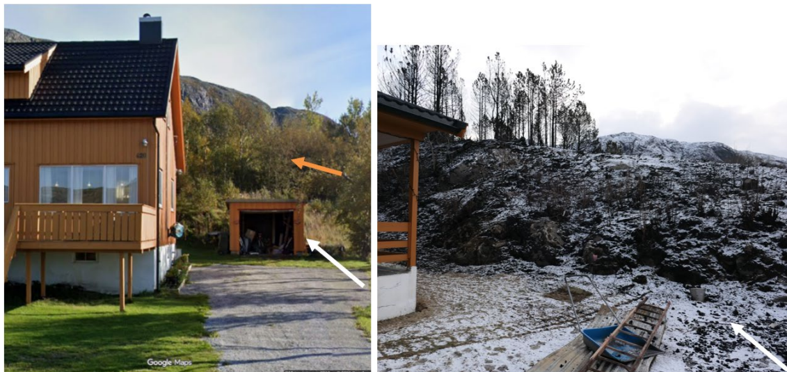
Figure A22. Before and after the fire, location 6. Garage 6a burnt down (white arrow). The tall vegetation marked by orange arrow has been cut down after the left image was taken, as can be seen in the post-fire photo to the right. Photo left: Google Street View (September 2019) ©2026 Google. Photo right: RISE Fire Research.
